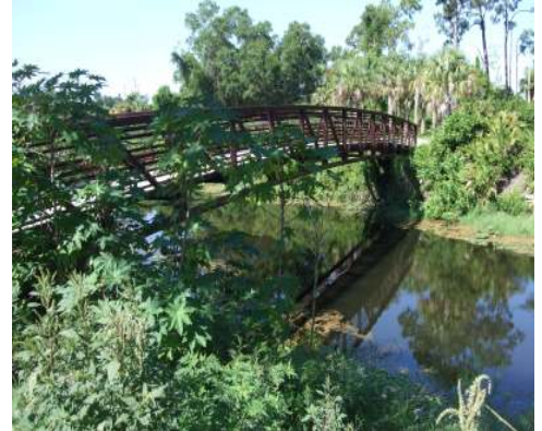
Steel Bridge outside our back gate (shown) will be closed going northbound.
