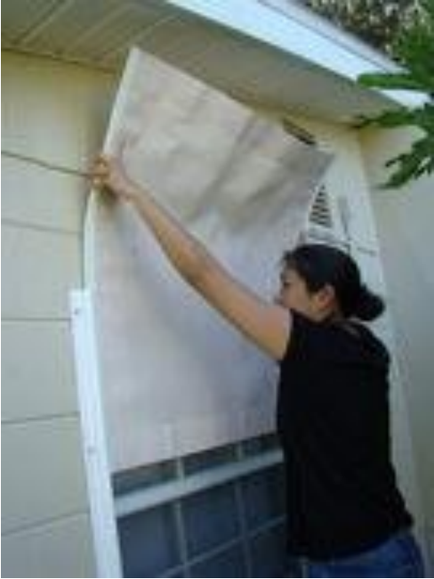
Storm Catcher Screen being applied
