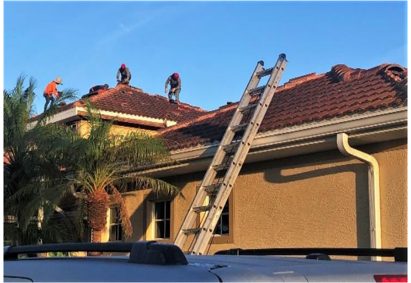
8:00 A.M. – October 24, 2023 The "strip-off" begins at 13861/63 Bently Circle
